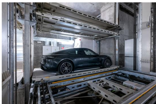
Image 3: The parking pallet is stored together with the car in a free parking space.
