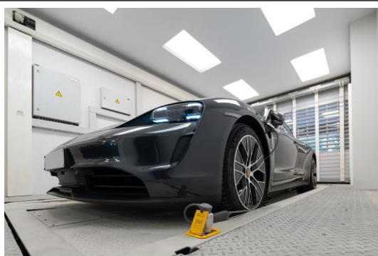
Image 1: Transfer cabin of the Multiparker 740. From here, the car is stored fully automatically.
