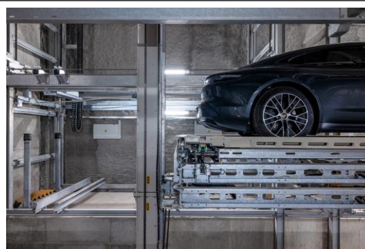
Image 2: The shuttle transports the car to its parking spot.
