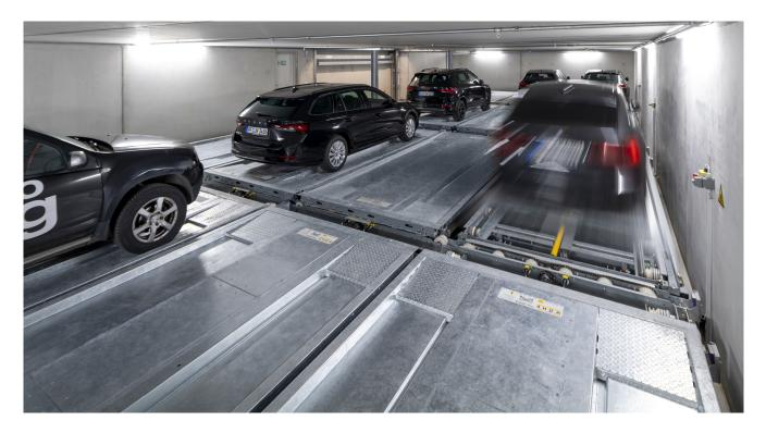
In the fully automated system Level Parker 570 cars are slided and glided closer together in a way like a puzzle. Flexible configuration options.
